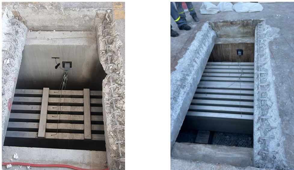
Figure 6. Tunnel sidewalls not damaged. Left – Potline 9, right – Potline 7 long tunnel. Both show busbar temperature monitoring thermocouples discussed later.
